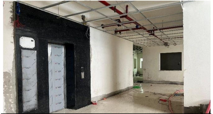
Photographs of progress August 2022
